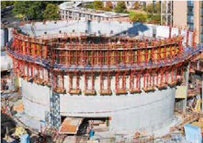
RUNDFLEX also for architectural concrete: depending on requirements, the very best surface qualities can also be achieved with the circular formwork.
