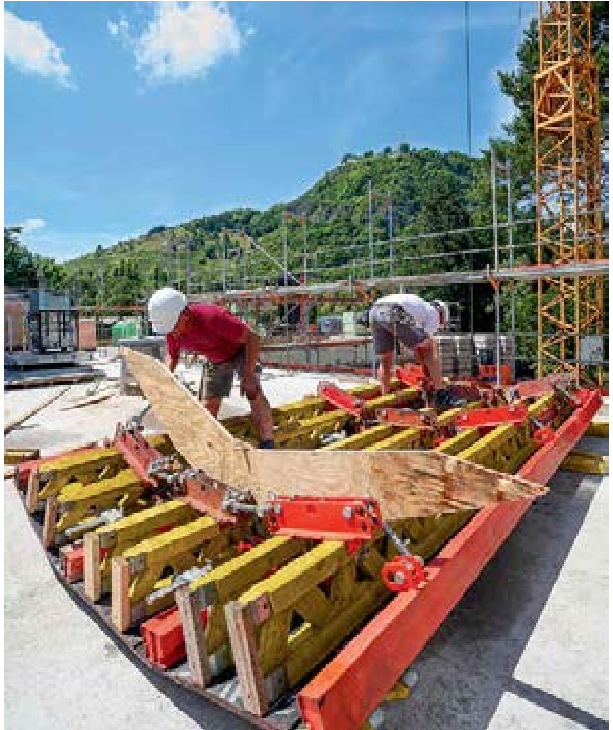
Checking the required curvatures is carried out by placing the radius template on the formwork girders.
