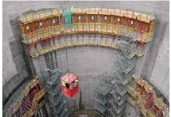
RUNDFLEX in use for the shaft of a pump station with a diameter of 25 m.
