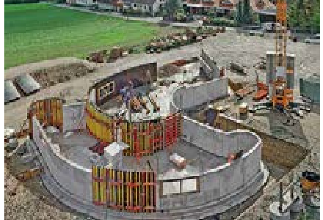
Exceptional challenge in housing construction: reinforced concrete walls with constantly changing radii and offset residential floors.
