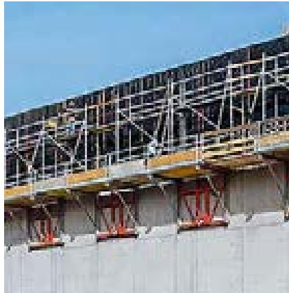
The folding corner platform on a straight wall section with vertically positioned PERI UP Reinforcement Scaffolding.
